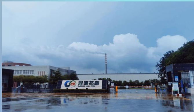
Guangdong Guanhao High-Tech annual of 300,000 tons of board paper replace project 广东冠豪高新年产30万吨板纸搬迁项目
